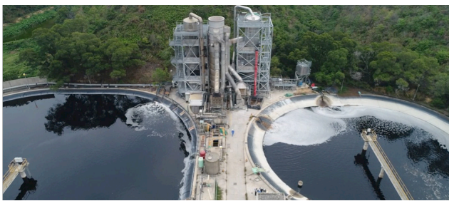
Figure 2. NENT landfill – 2500 m 3 /hour.
